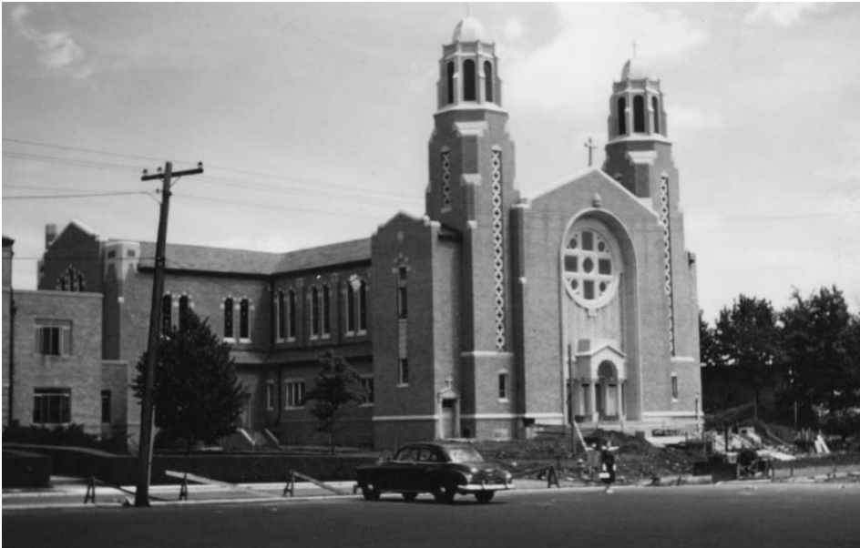
▲ St. Thomas under going final construction. The first mass said in the current church was February 21, 1960.
